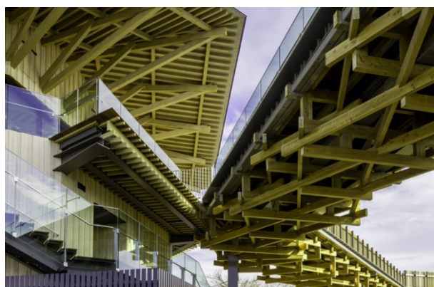
Fig.13 Combination of Steel and Wood in Nihondaira Yume Terrace
