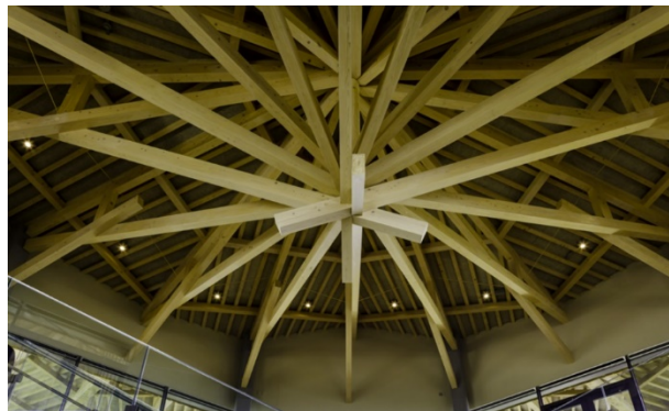
Fig.12 Distorted Mortise-and-Tenon Joints of Nihondaira Yume Terrace
